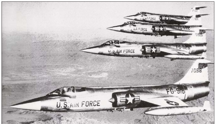
The Lockheed F-104C “Starfighter” is shown above. The 83d had the F-104A whose thin 22 foot straight wing in the era of swept wings could carry the 23,000 pound plane at speeds up to 1,300 MPH.
