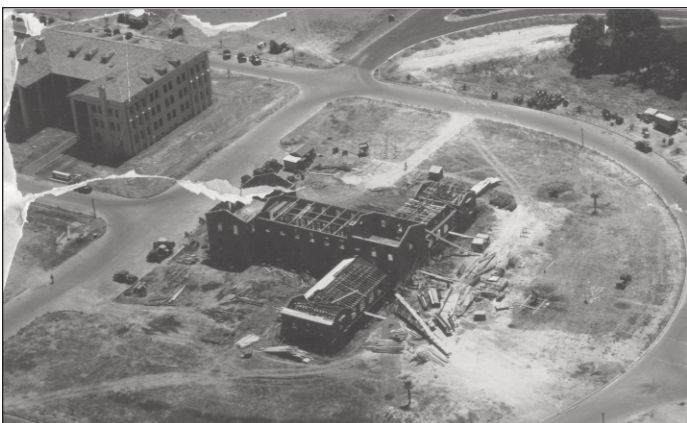
Headquarters building—left top Air Corps barracks #420 completed October 26, 1934 at a cost of $149,301.
