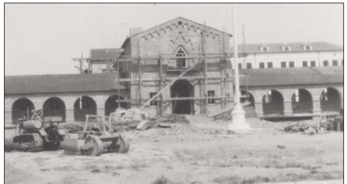
Construction of Headquarters Building, building #500, completed November 16, 1934 at a cost of $82,292.
