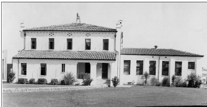
Picture of Fire and Guard house on Nov. 2, 1937. The Fire house was completed August 18, 1934 at a cost of $37,799. The fire house is now without the 3-cell brig.
