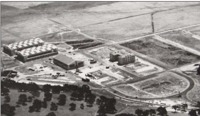
Construction of Hamilton Field on July 15, 1933.
