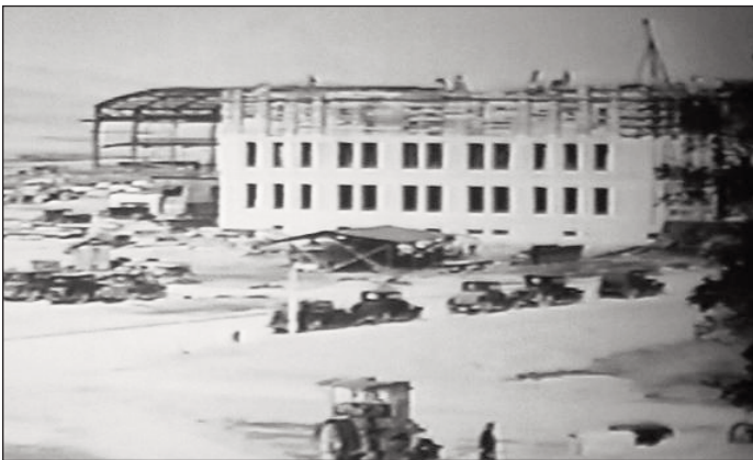
Construction of the first barrack #422, completed July 31, 1933 at a cost of $131,644. Hangars 8 and 9 under construction in the background. (Pictures taken from the Hamilton Story "Mission Completed." DVD for sale at the museum.)
