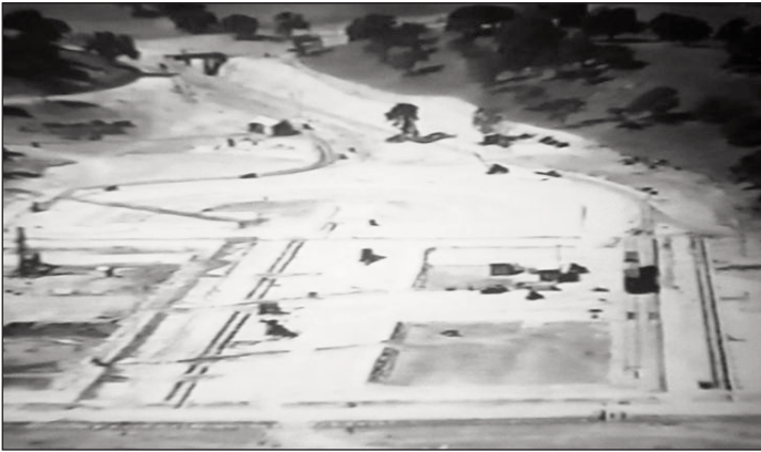
Railroad spur track on far right was completed September 9, 1932 at a cost of $19,395.
