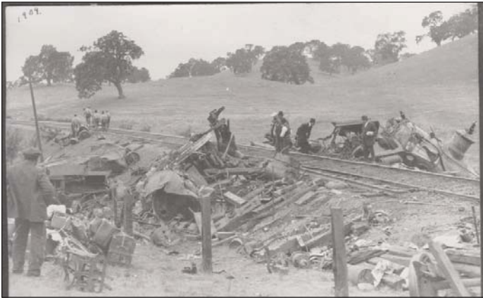
The heap of wreckage was piled high along the sides of the track, and the torn, sprung tracks were straightened and made firm for resumption of traffic by the morning.
