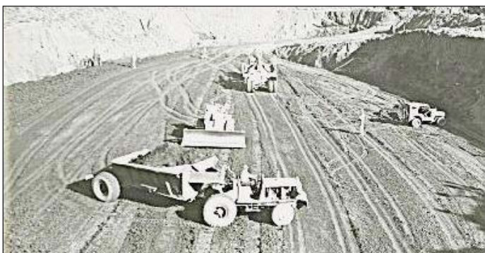
Bulldozers and carryalls dig into the bed of Novato Creek in construction of the dam.
