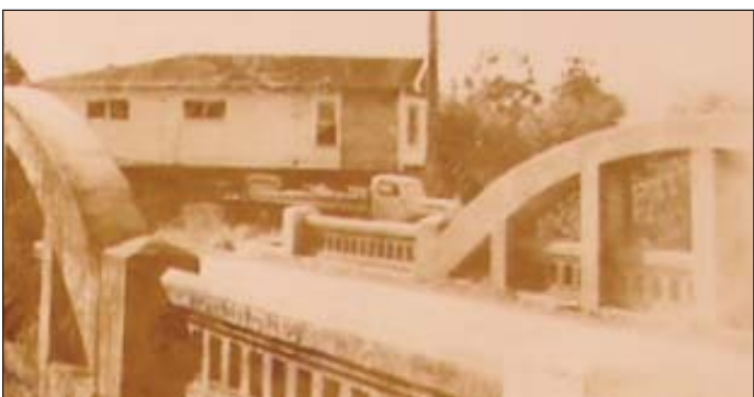
Photo of the Grossi home, which was moved from First Street to the Grossi ranch next to Stafford Lake. Here the house is about to cross the Novato Blvd. bridge.
