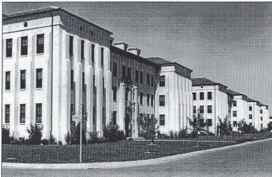
The enlisted personnel barracks circa 1940. This particular area has been preserved and looks the same in 2006.
