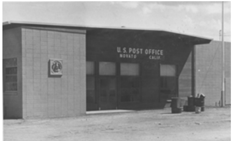
Post Office #7: First Street Post Office now Don Johnson's Pool
