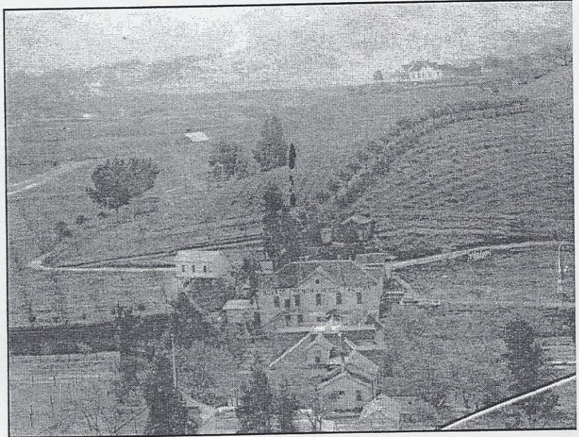
The Novato French Cheese Co., formerly the California Creamery Co. is in the foreground. The row of olive trees, leading up the hill, in the center of the photograph are on Theodore Reicherts' property and are standing to this day. The Daniel Hayden residence is visible at the top of the hill in the distance.
