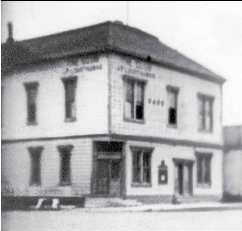
John P. Loustaunau would have the porch removed and add concrete sidewalks in May of 1923.
