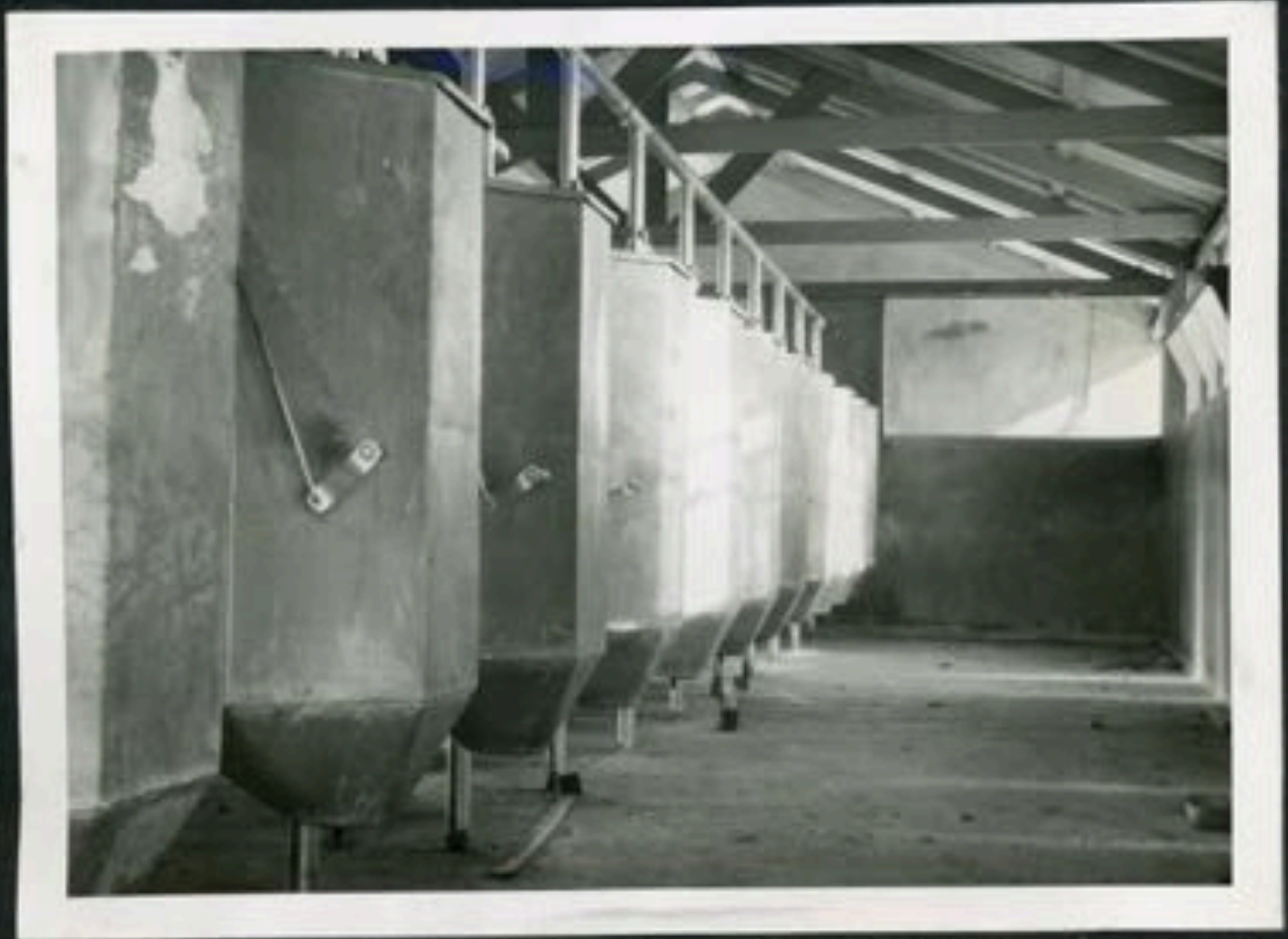
REAR VIEW OF FEED MANAGERS WALK THROUGH UNIT.
