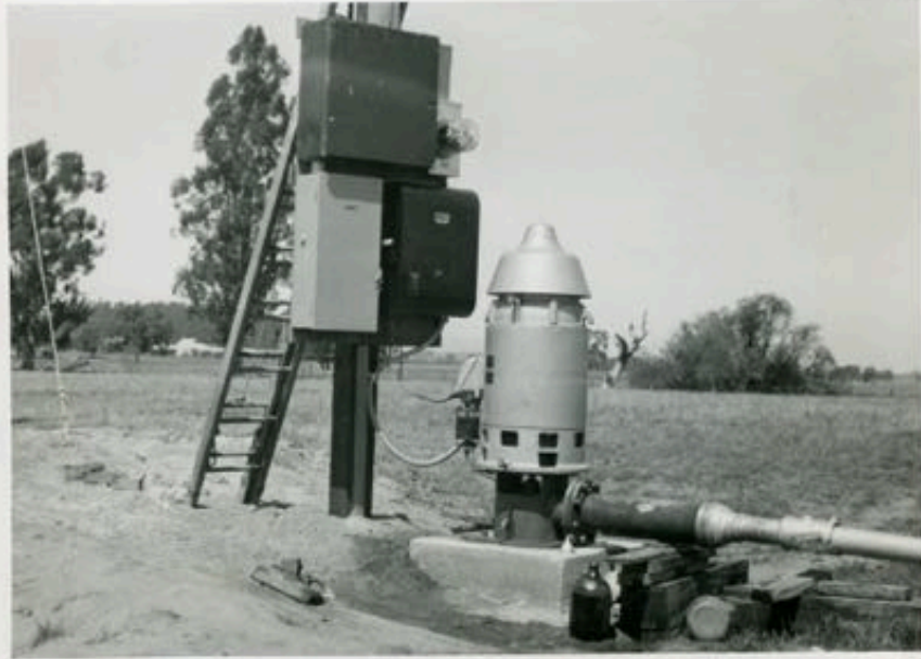
ARTESIAN WELL AND FORTY H.P. ELECTRIC MOTOR PUMPING 800 GALLONS PER MINUTE AND SUPPLYING 32 SPRINKLERS IN SONOMA CO.
