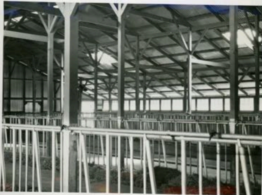
INTERIOR VIEW OF A STEEL STANCHION MILKING UNIT
