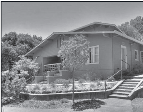
Picture of the Parkhaven clubhouse
