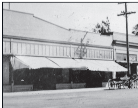
Picture of the building in 1917
