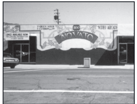
Picture of the building in 1970
