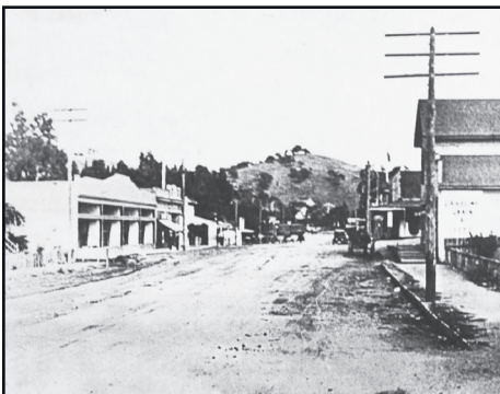
Picture of the building in 1916
