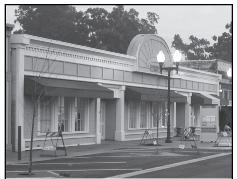
Picture of the building in 2004
