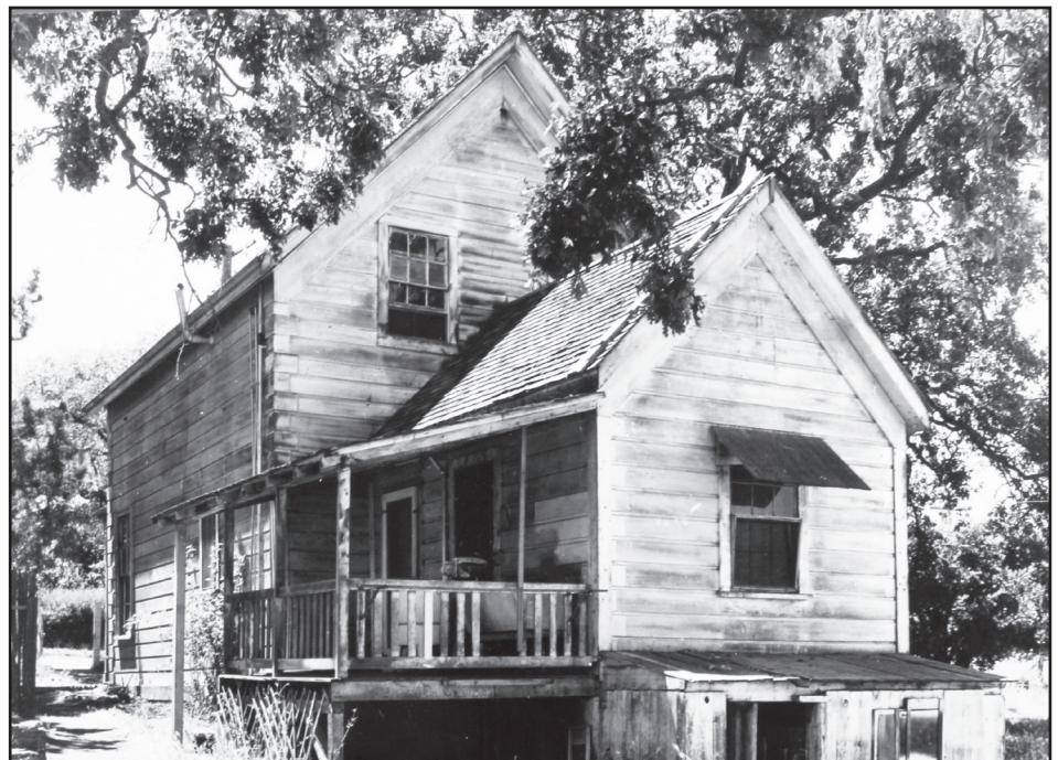
Back view of the Clark house in Novato built by the Pachecos shows its architectural grace and kinship to New England.
