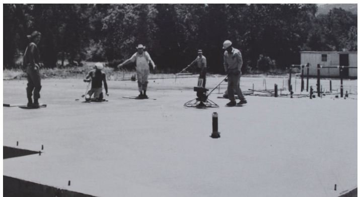
July 3, 1974—Floor slab had been poured
