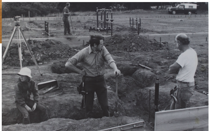
June 5, 1974—Dave Milano in the trenches
