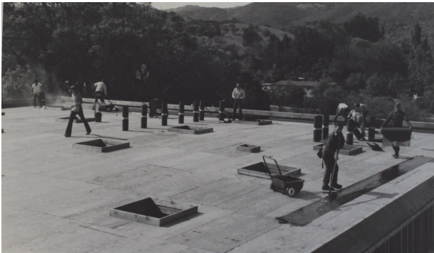
May 7, 1975 gymnasium roof getting tarred and graveled
