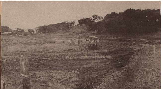
Grading started at the Olive Ridge Tennis Club site off Olive Avenue. Tennis courts and parking will be provided in the flat area in front of the low ridge (in the back ground which will contain later a 5000-seat stadium for major West Coast tennis tournaments and clubhouse.
