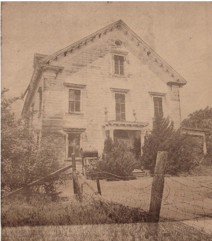
View of the late Robert H. Trumbull's "Home Place" Rancho Novato showing an unused doorway once the carriage entrance to a hallway between the front and back parlors. A long circle driveway swept past this doorway during the height of Novato Rancho's wealth and prosperity in the 1870's and 1880's. Distinguished persons drove fine equipages followed by coach hounds.
