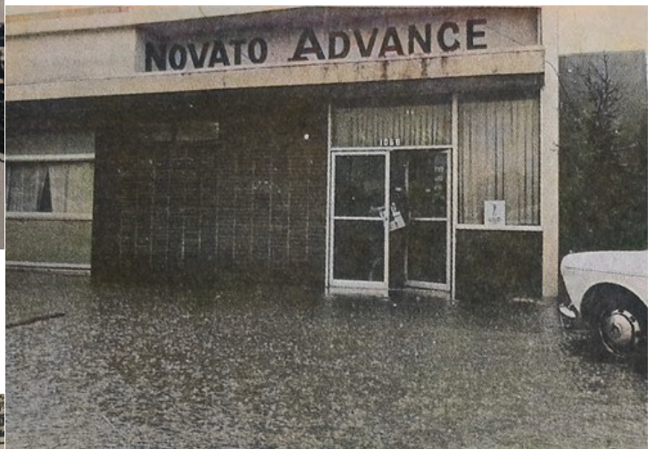
“Water lapped at the doors of the Novato Advance during the heavy squall that flooded intersections and swamped the city's overloaded drainage system. A passing truck sent a wave to splash under the doors of the Advance. Water entered the editorial department. If some of the stories in the Advance appear to be all wet, blame the weather. Some 1.82 inches of water fell yesterday, bringing the season's total to 40.95 inches. However due to a lack of high tides, creeks did not overflow their banks.”
