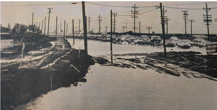
“Southbound drivers on U.S. Highway 101 would have made their pioneer forebearers proud when they successfully navigated a flooded section of Highway 101 near the Sportsman Lodge. The traffic backed up as far as Rancho Olompali, as cars moved slowly toward the flooded area and then, like covered wagons, forded the shallow river.”
