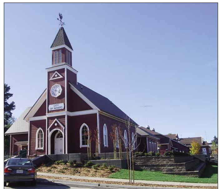
Our new/old city hall showing the new patio, retaining wall, benches and part of the lawn area on the north side of the building.
