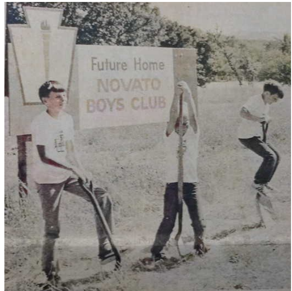
Groundbreaking ‘rehearsal’ - Novato Boys’ Club members Tom Cox, Dan Milano and Scot Eustace found out that groundbreaking is a backbreaking job this time of year when they rehearsed for the public ceremony at 680 Wilson Avenue.
